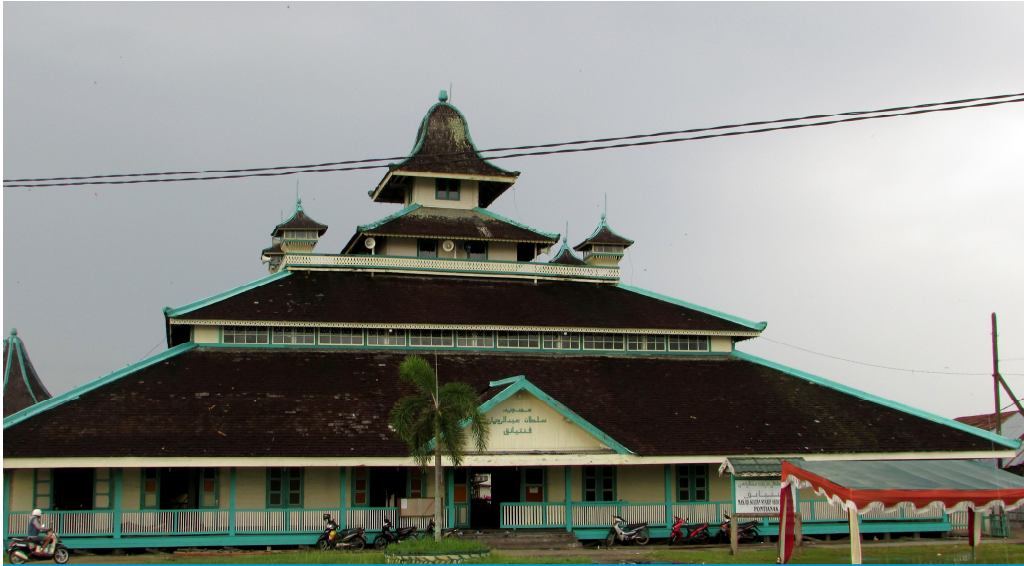
Picture 2: Jami' Sultan Abdurrahman mosque in Pontianak. Its building process started in 1821. The building size is 33,27 m x 27,74 m
